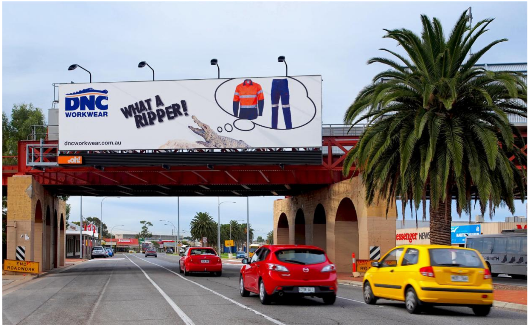
SA, Port Adelaide, Commercial Rd Bridge
